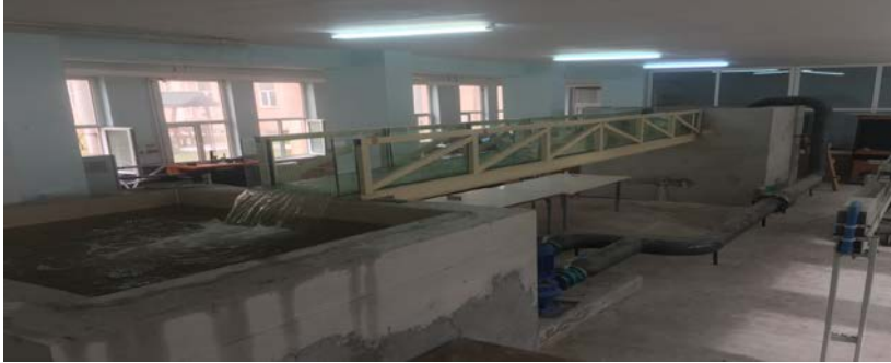
Figure 5. General view of the open channel system
