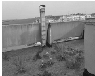
Figure 4. Roof in Ruse, Bulgaria
