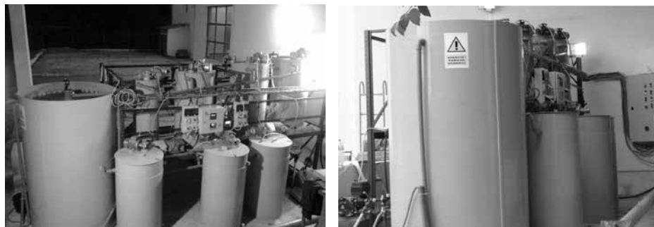
Fig. 2. ECOIND HDS pilot plant in operation at Alunis-IIba
