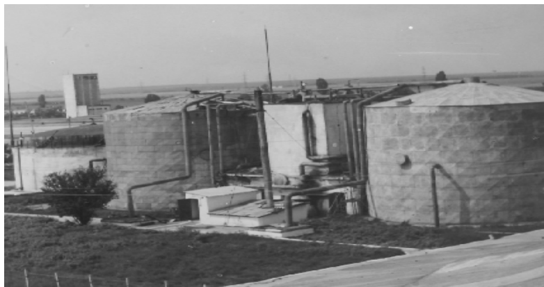
Fig 3. Caracal anaerobic treatment plant made of metal with biogas production, capacity 4 \times 1200\text{m}^3 [10.]
